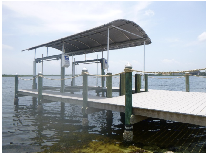
Photo 6: Facing Southeast, view of dock and covered canopy.
